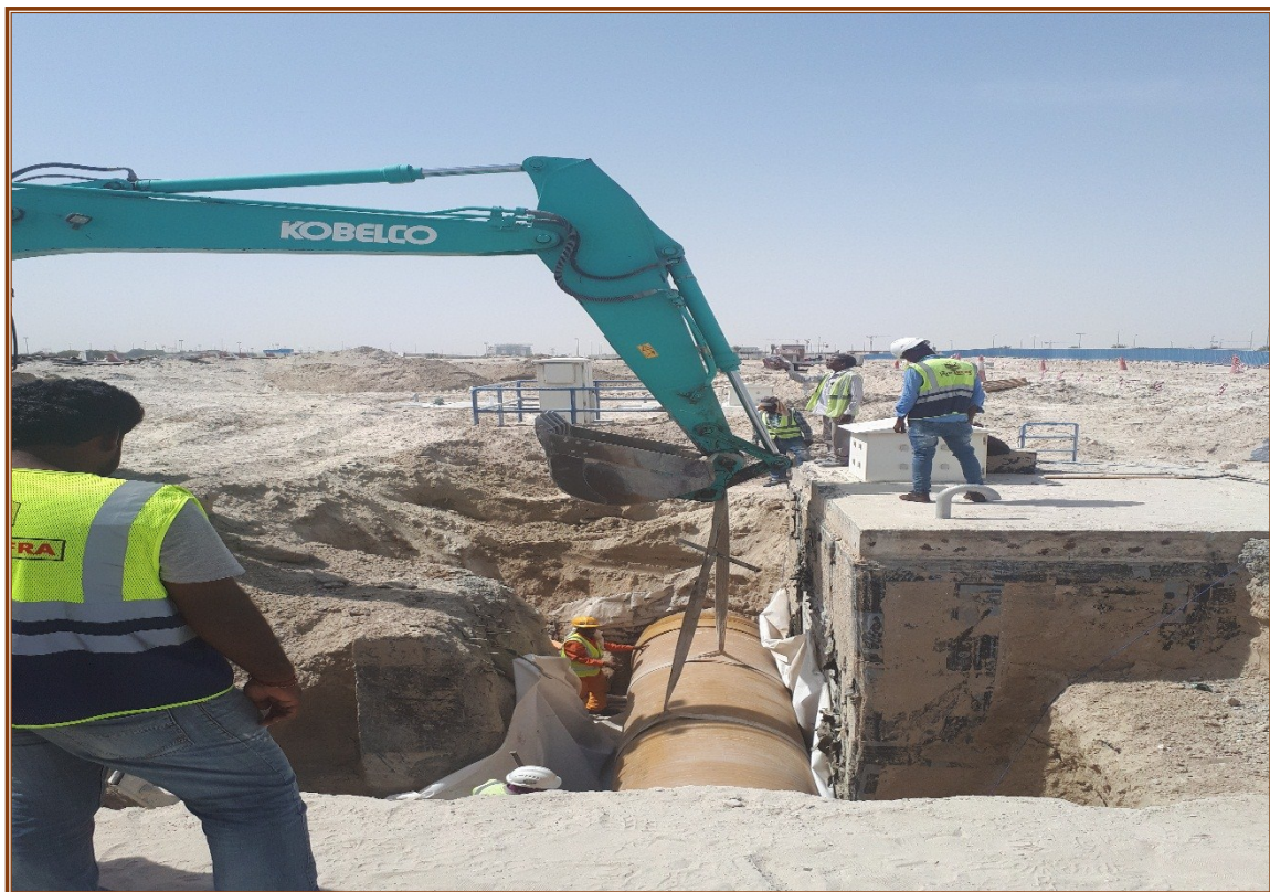
DIA1200mm SHUTDOWN WORK AT DUBAI DESIGN DISTRICT
