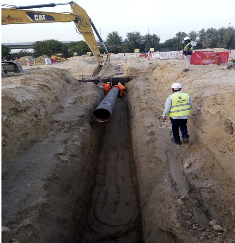
DIA610mm STEEL SLEEVE PASSING UNDER 132kv TROUGH IN SOBHA HARDLAND AT MBR CITY
