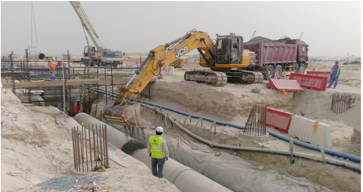
LAYING OF 1100mm dia DRAINAGE WORK AT DP WORLD JAFZA
