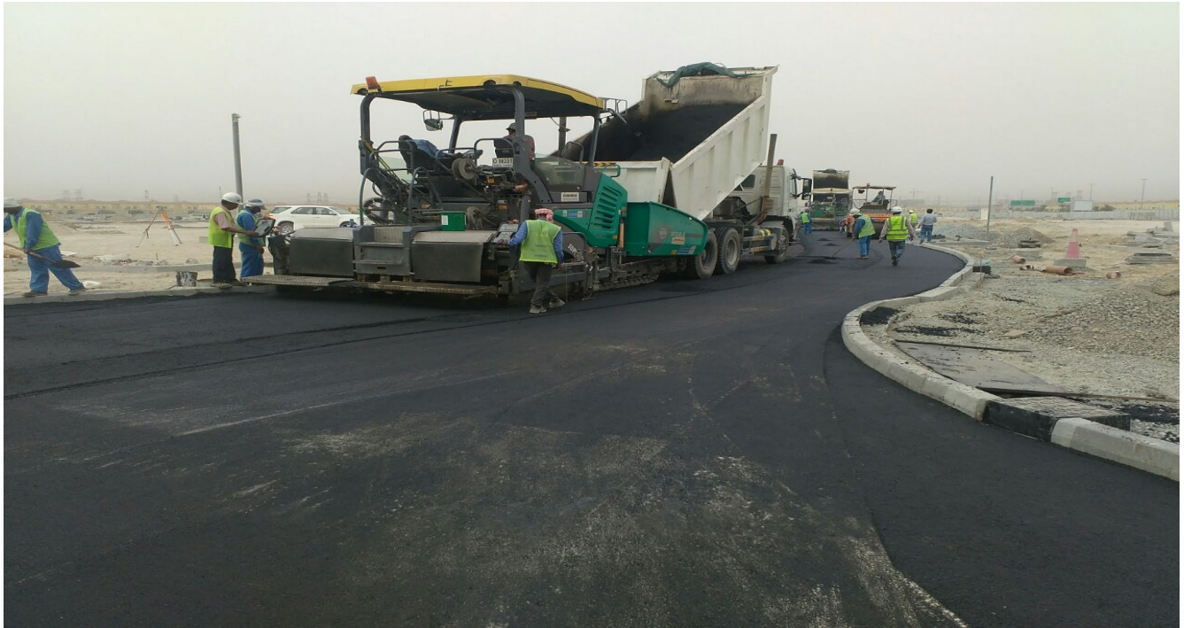
ASPHALT LAYING AT JUMEIRAH PARK
