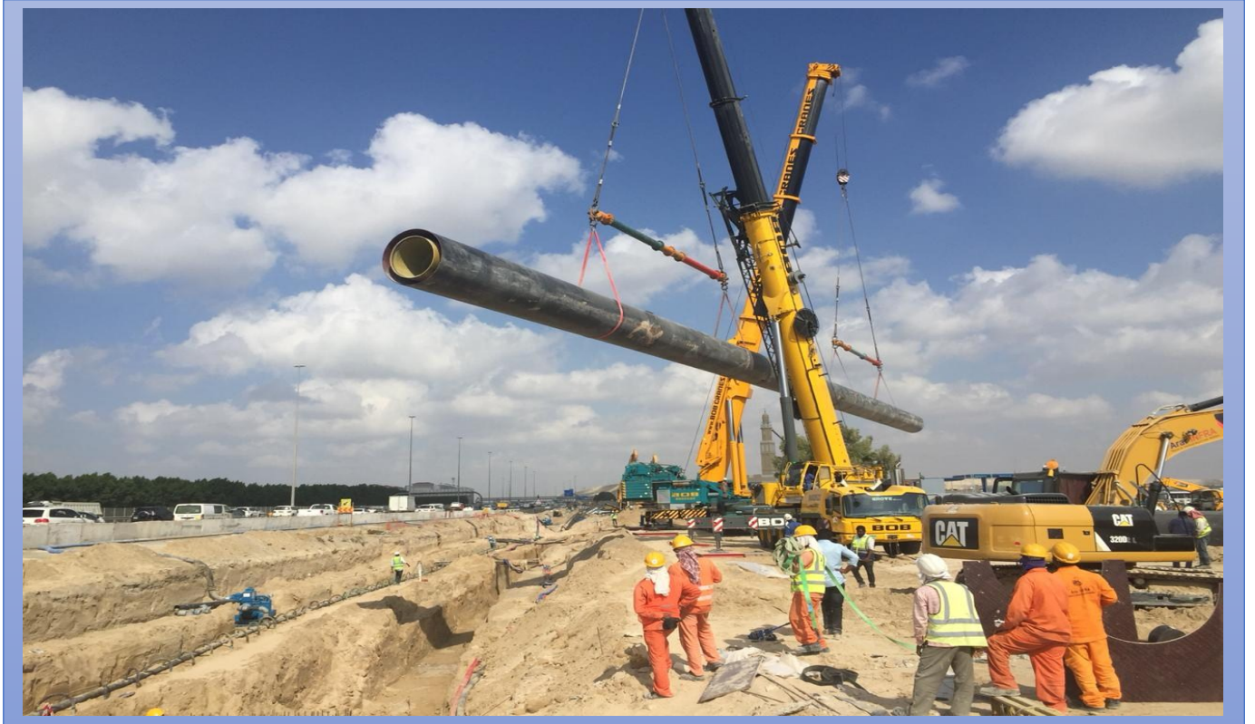
1200mm STEEL SLEEVE PROTECTION AT MUHAISNAH
