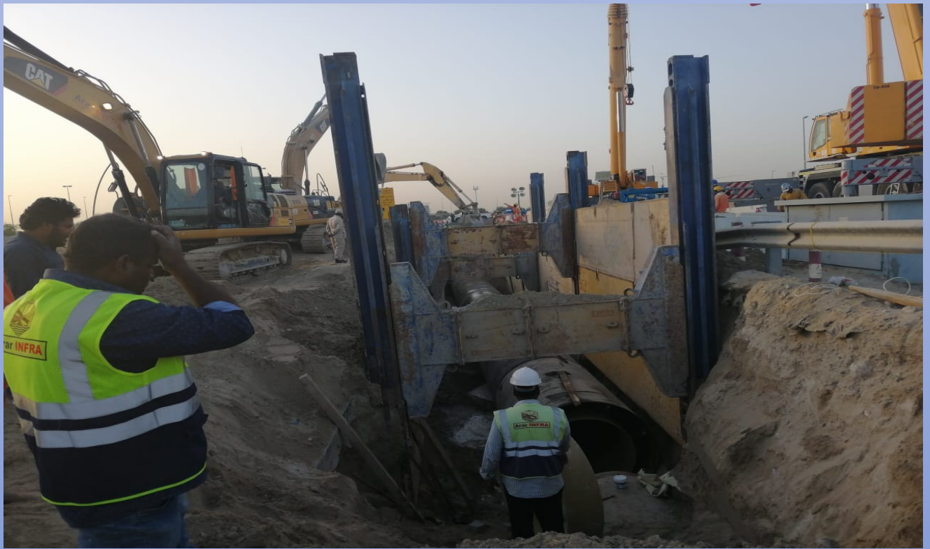
1200mm STEEL SLEEVE PROTECTION AT DESIGN DISTRICT
