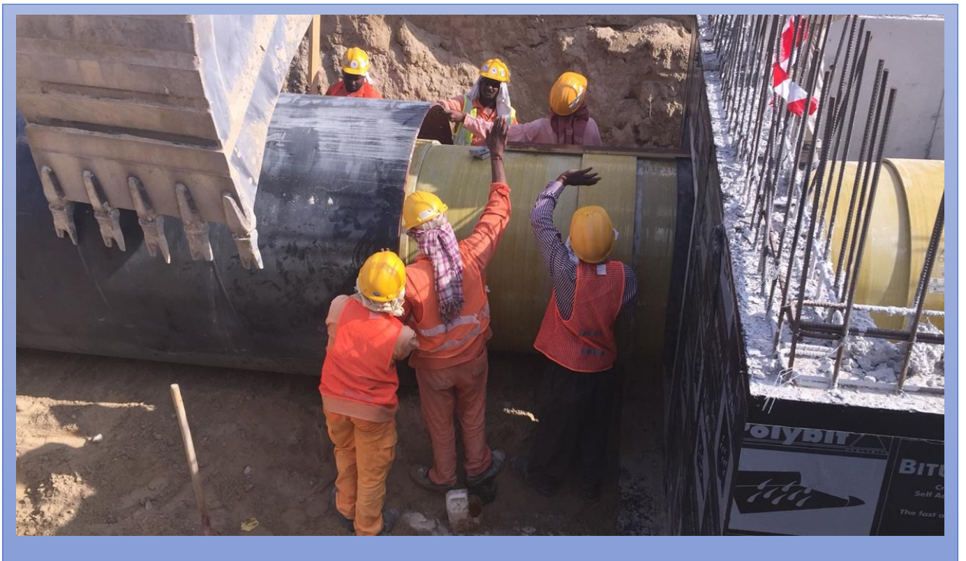
1200mm STEEL SLEEVE PROTECTION AT MUHAISNAH
