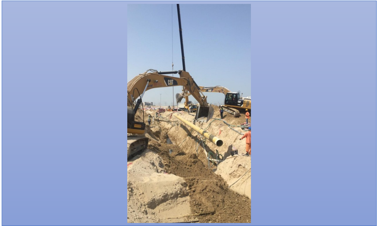
600mm GRE PIPE INSTALLATION AT GEMS SCHOOLS AL BARSHA
