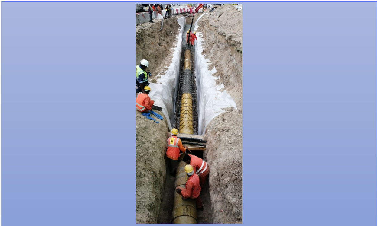
600mm GRE PIPE PROTECTION AT R1015/3B AL SZRD
