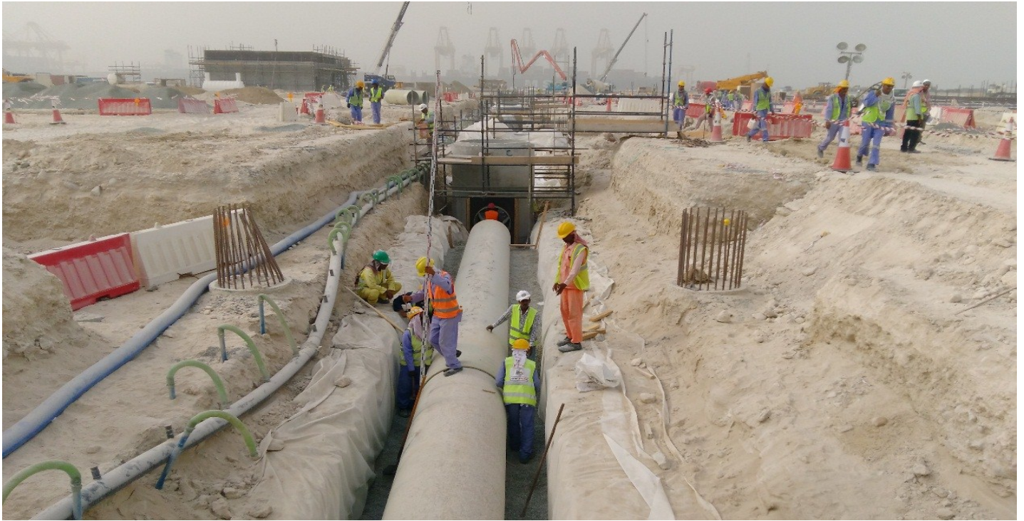
LAYING OF 1100mm dia DRAINAGE WORK AT DP WORLD JAFZA
