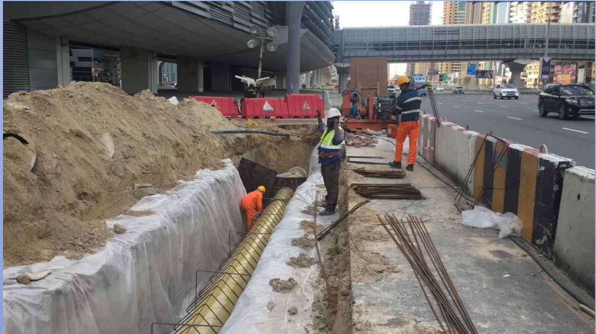
600mm GRE PIPE INSTALLATION AT R1015/3B AL SZRD
