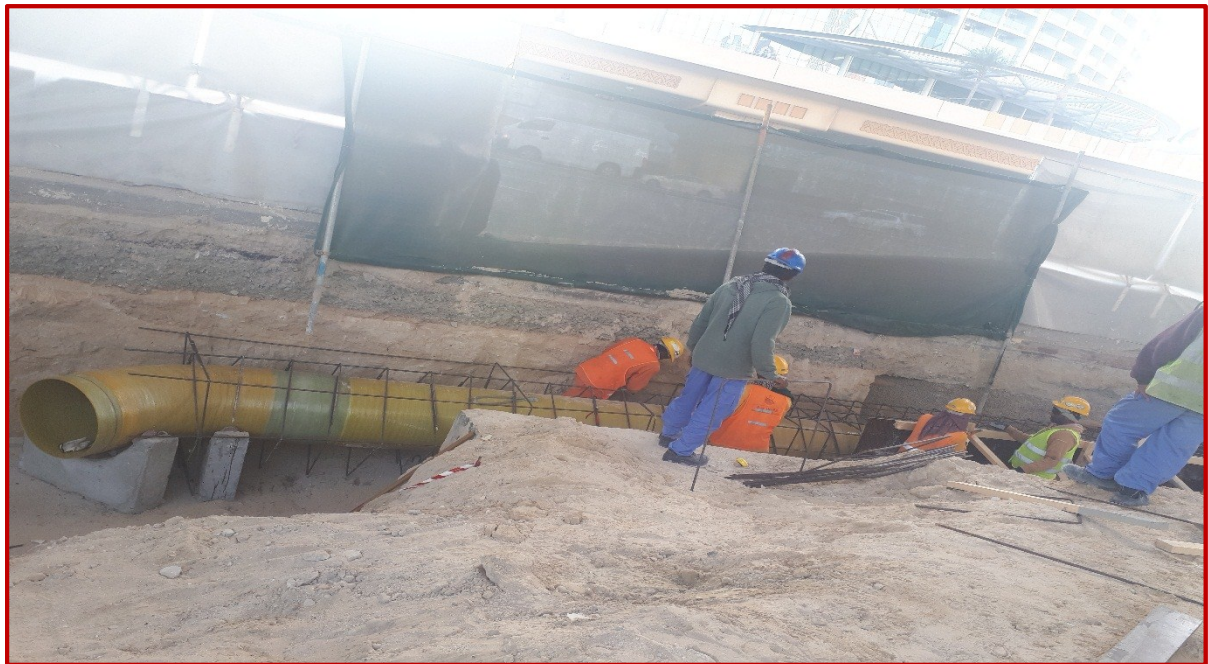
DIA600mm SHUTDOWN WORK THE DUBAI MALL –ZABEEL CAR PARK EXPENSION
