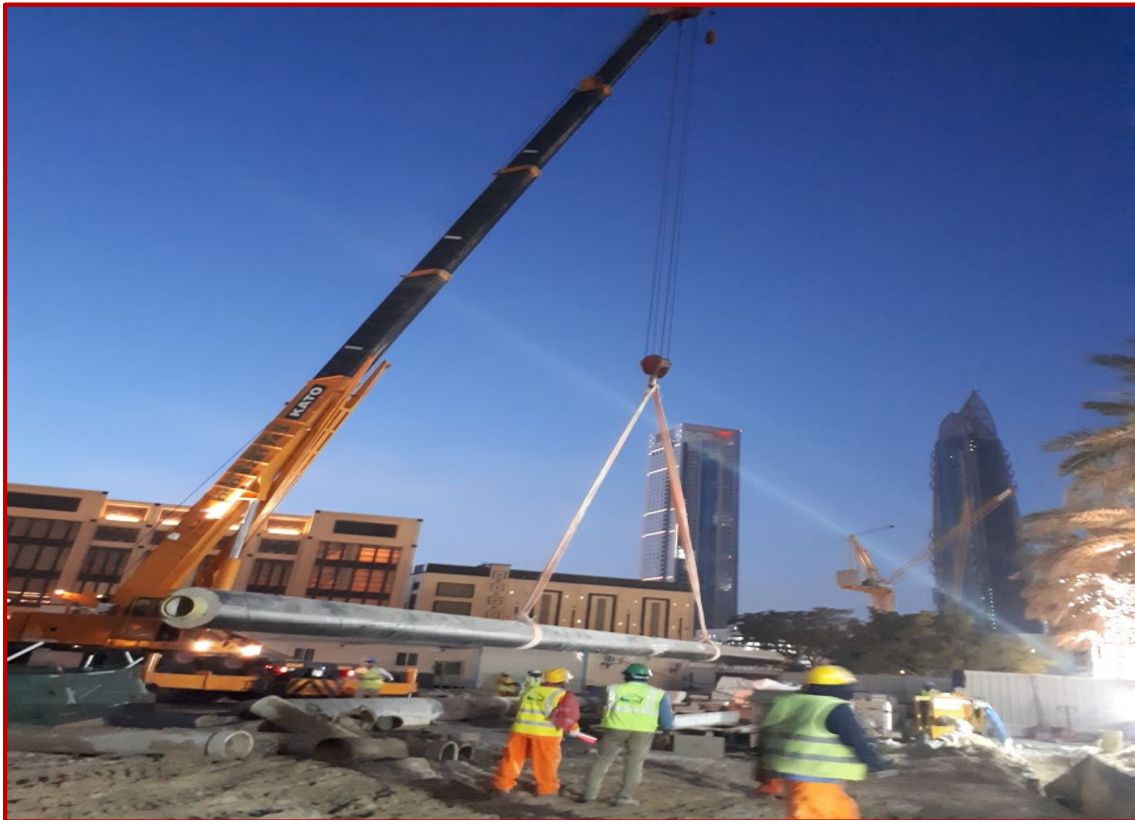
DIA600mm PIPE SHUTDOWN WORK AT DUBAI CREEK HARBOUR
