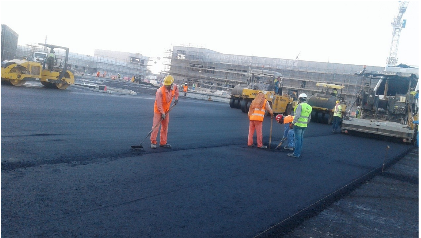
ASPHALT LAYING AT LEGOLAND
