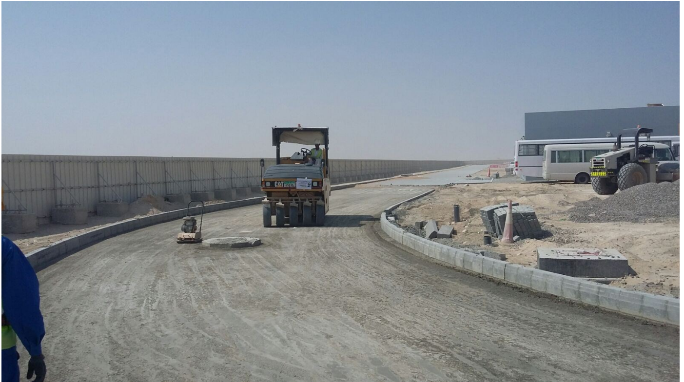
SUB BASE PREPARATION AT DUBAI PARK (LEGO LAND)
