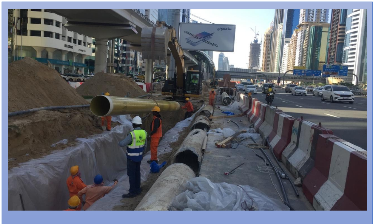
600mm GRE PIPE INSTALLATION AT R1015/3B AL SZRD
