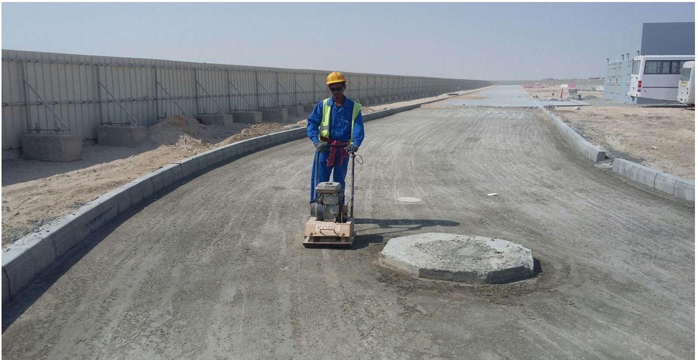
SUB BASE PREPARATION AT DUBAI PARK (LEGO LAND)
