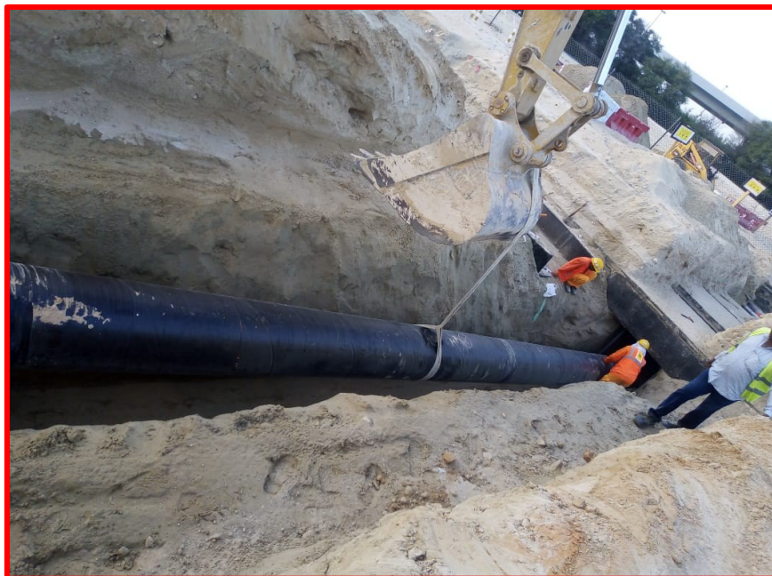
DIA610mm STEEL SLEEVE PASSING UNDER 132kv TROUGH IN SOBHA HARDLAND AT MBR CITY
