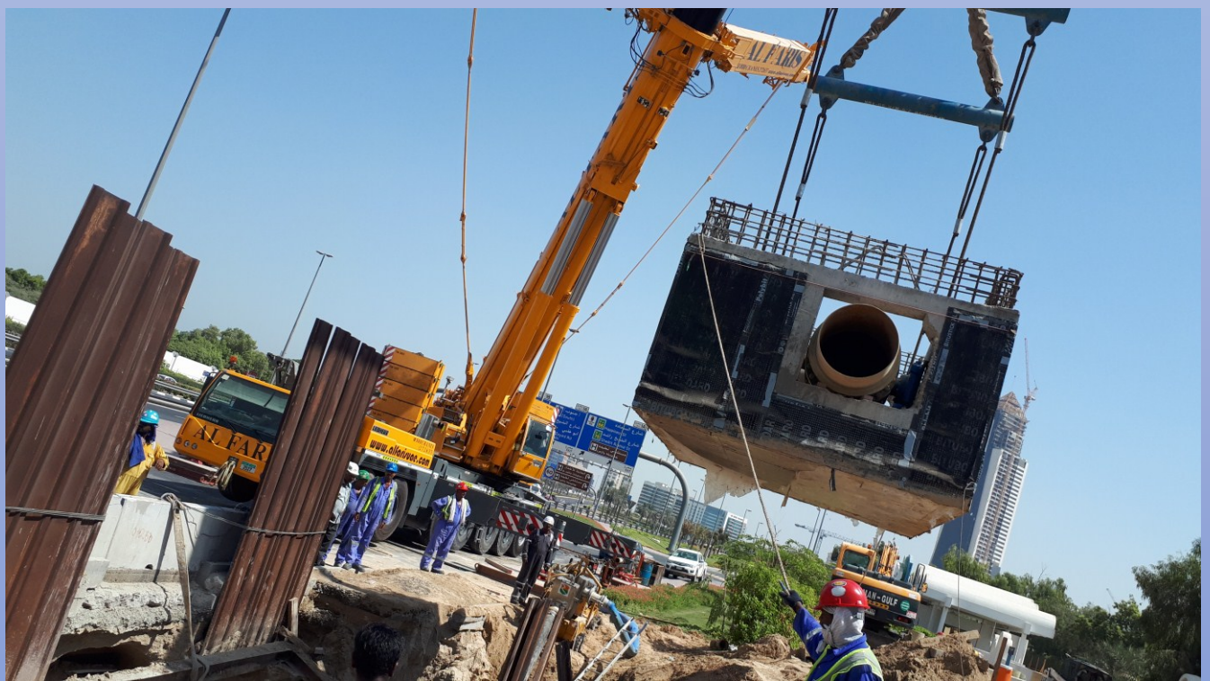
500mm DIA IRRIGATION CHAMBER AT LATIFA HOSPITAL
