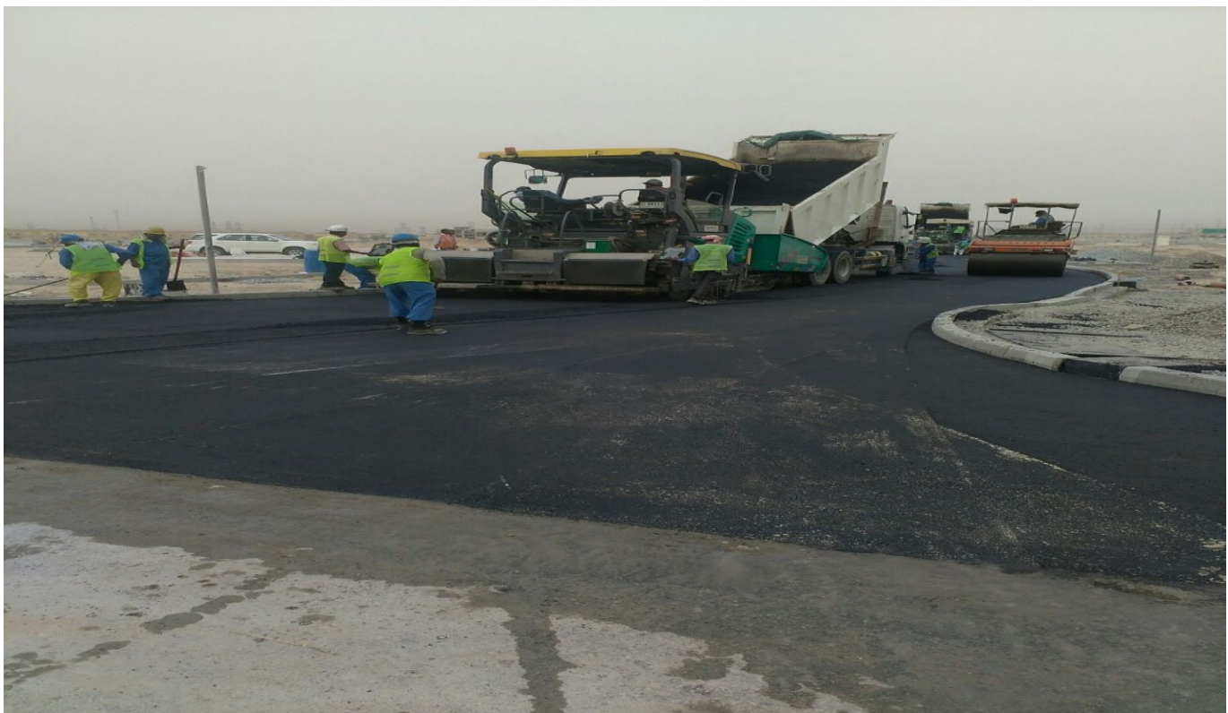
ASPHALT LAYING AT JUMEIRAH PARK
