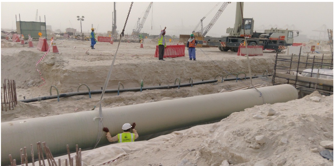
LAYING OF 1100mm dia DRAINAGE WORK AT DP WORLD JAFZA
