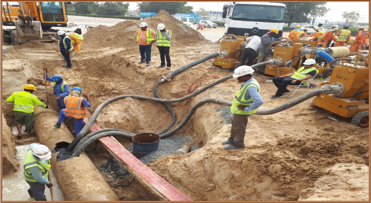
DIA600mm PIPE SHUTDOWN WORK AT DUBAI CREEK HARBOUR
