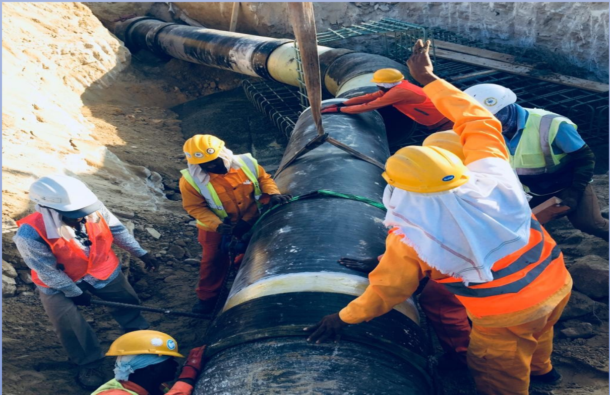
800mm DIA IRRIGATION PIPE
