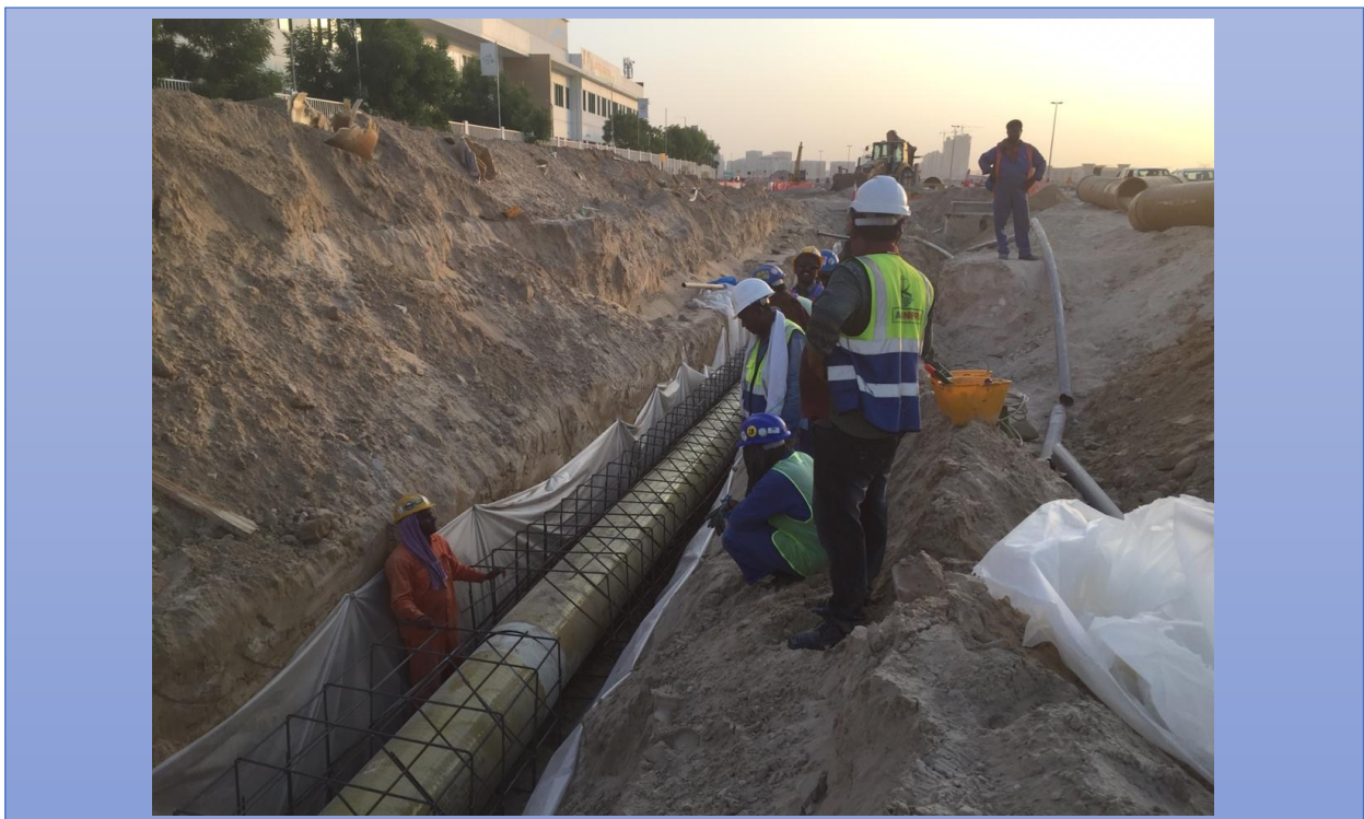
600mm DIA PROTECTION AT GEMS SCOOOL AL BARSHA
