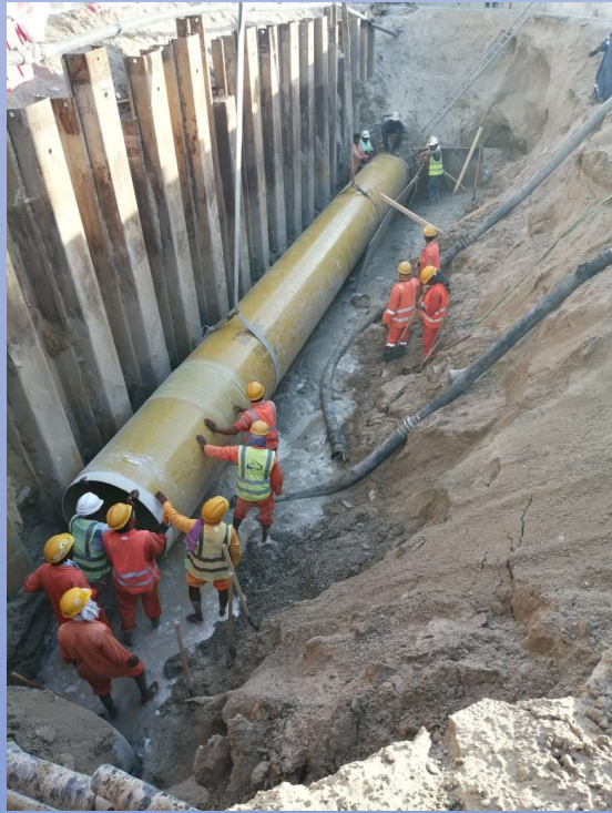
1200mm GRE PIPE PROTECTION AT R1015/3B AL SZRD
