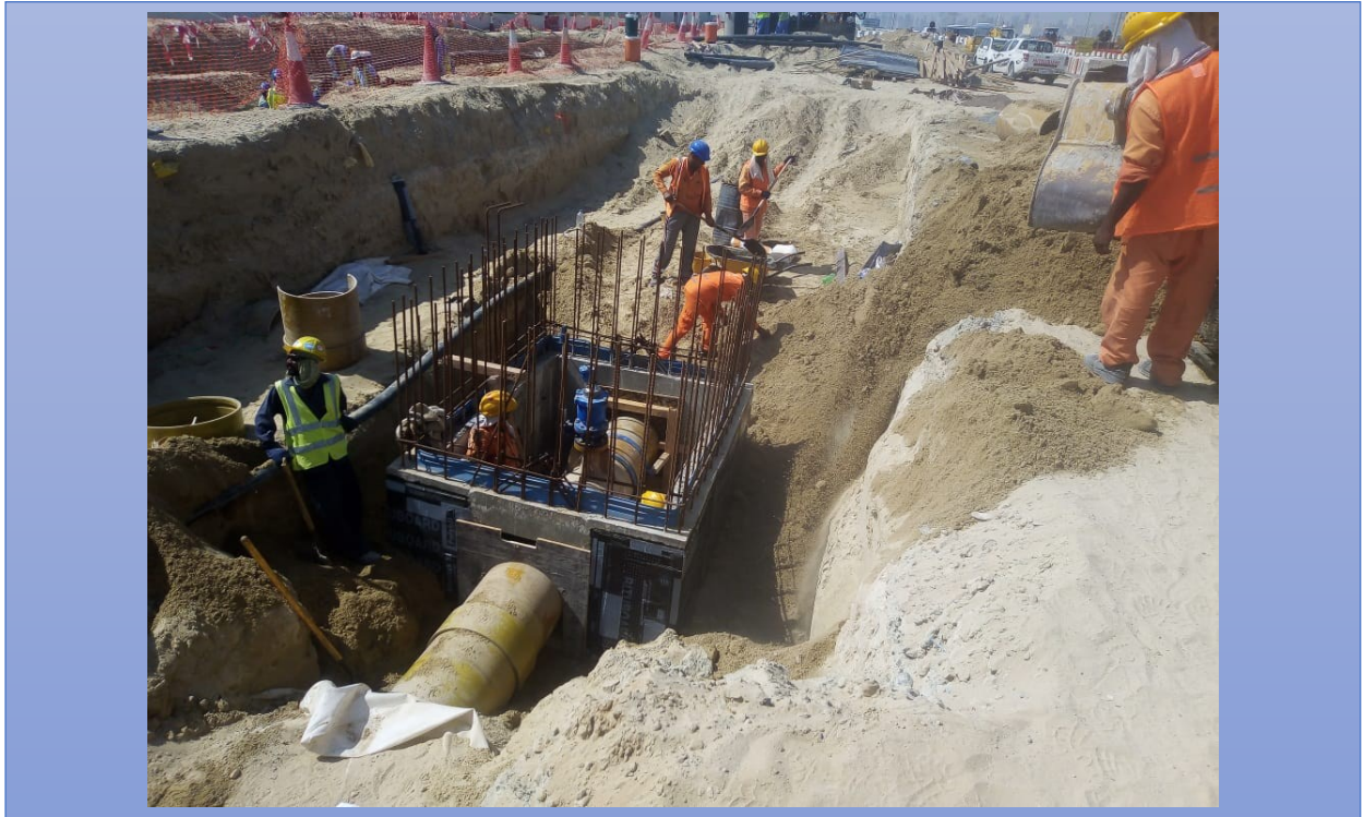
AIR VALVE CHAMBER INSTALLATION AT GEMS SCOOOL AL BARSHA
